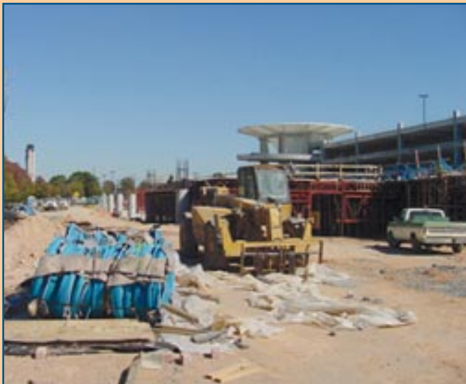
New parking garage construction
