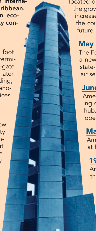
The air traffic control tower at RDU is responsible for air space within approximately 40 miles of the airport and up to 10,000 feet above ground level.
