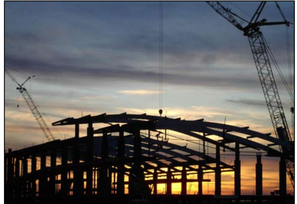
Major construction on RDU's Terminal 2 began in the spring of 2006.
